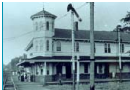
The Canaan, CT railroad station
